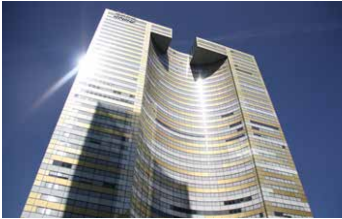
Tour Eqho - France - Clima Canal
