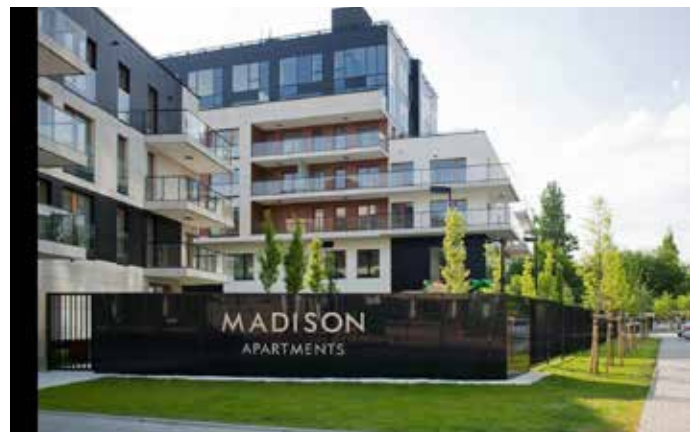
Madison Apartments - Poland - Clima Canal
